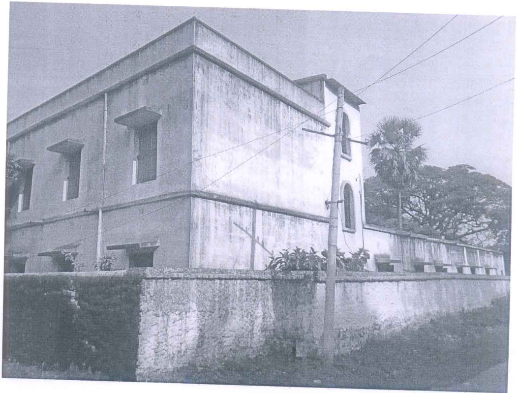
Rear view of the building
